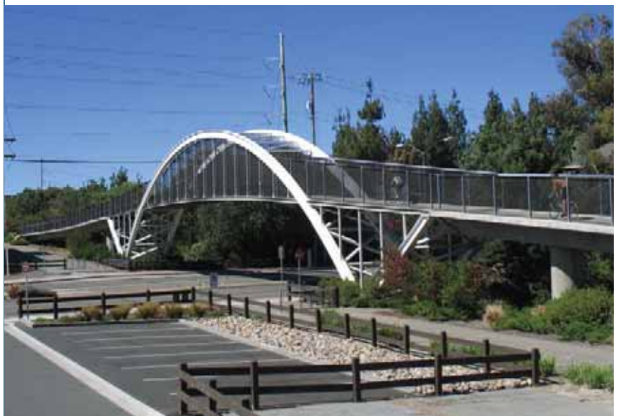
OVERCROSSING AT YGNACIO VALLEY ROAD
