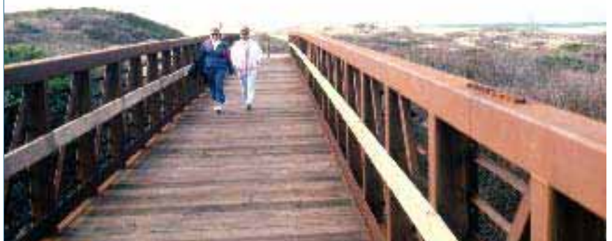
JOHN HERNANDEZ BRIDGE
