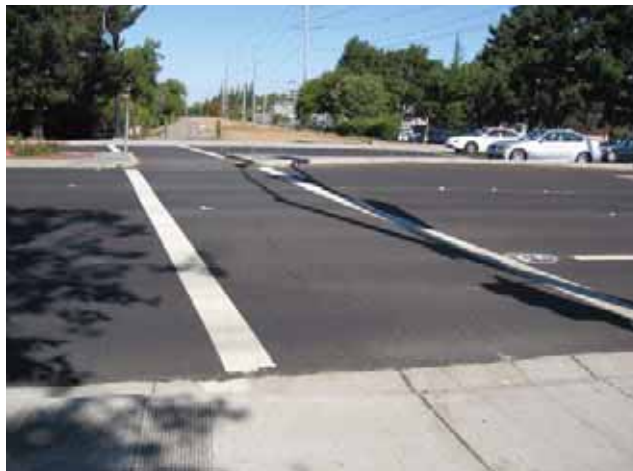
CROW CANYON ROAD CROSSING
